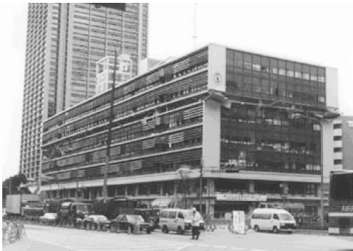
图 3 阪神地震某结构第 6 层破坏跨塌 Fig. 3 Collapse of the Sixth-story Structure in Kobe Earthquake
