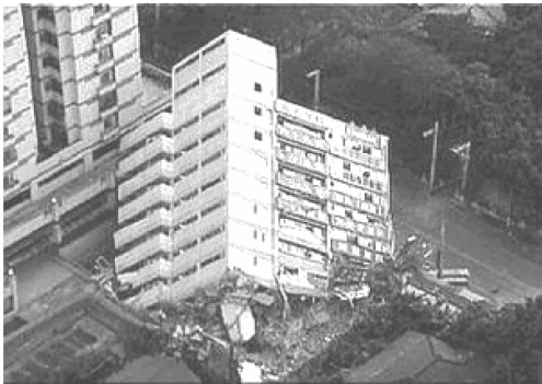
图 4 集集地震某结构底层破坏倒塌 Fig. 4 Collapse of Bottom Frame Structure in Chi-Chi Earthquake
