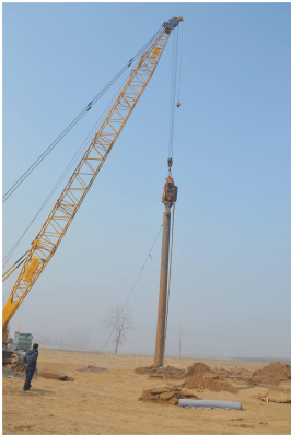
图 3 振动沉管施工现场 Fig. 3 Construction Site of Vibration Pipe Sinking
