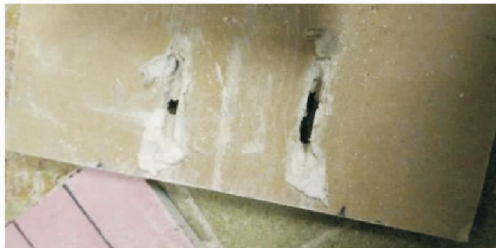
(c) 双层双面石膏板的背面长槽形缺口
