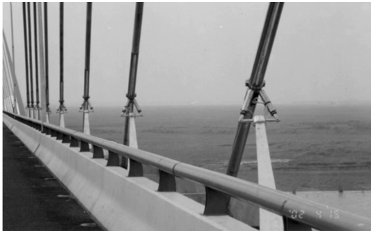
图 11 洞庭湖大桥拉索减振系统 Fig. 11 System of mitigating vibration of cables on Dongting Lake Bridge
