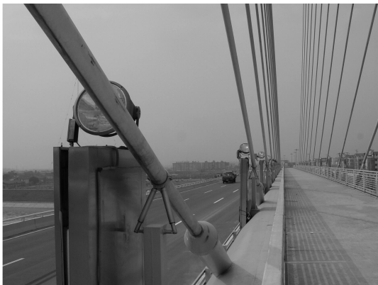
图 12 洪山庙大桥拉索减振系统 Fig. 12 System of mitigating vibration of cables on Hongshanmiao Bridge
