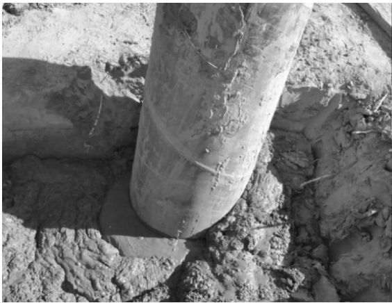
图 8 淤泥沿管壁外侧涌出地面 Fig. 8 Sludge Poured Out of Ground Along Outside of Pipe
