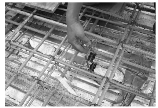
图 3 浇灌混凝土前在桥面板内埋设应变计 Fig. 3 Embedding of Strain Gauges in Deck Before Concrete Casting
