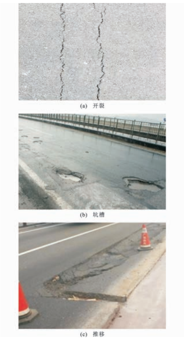
图 17 正交异性钢桥面沥青铺装层病害 Fig. 17 Damage Issues of Asphalt Pavement on Orthotropic Steel Deck
