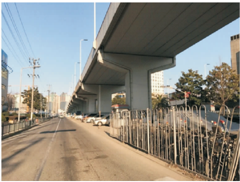
图 8 需整体降落的南侧八跨桥段 Fig. 8 Eight Segments Need Low Down at South of Bridge
