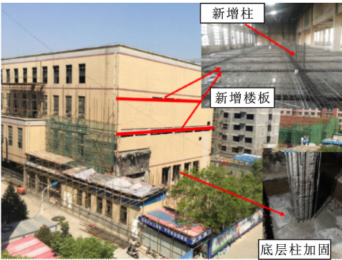
图 1 既有建筑增层基础加固照片 Fig. 1 Photos of Foundation Reinforcement of Existing Building
