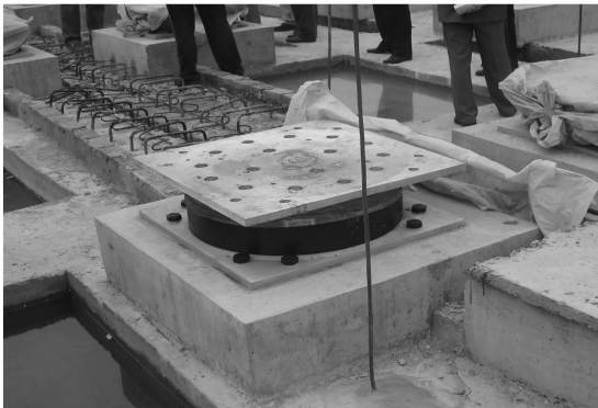
Fig. 2 Installation of Isolation Rubber Bearing 图 2 橡胶隔震支座安装
