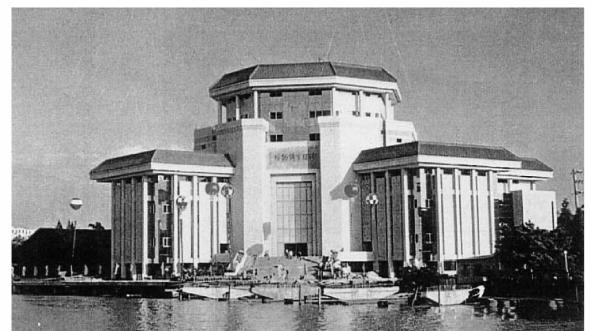
Fig. 7 RC Frame-Shear 13 Stories Museum with Story Isolation
